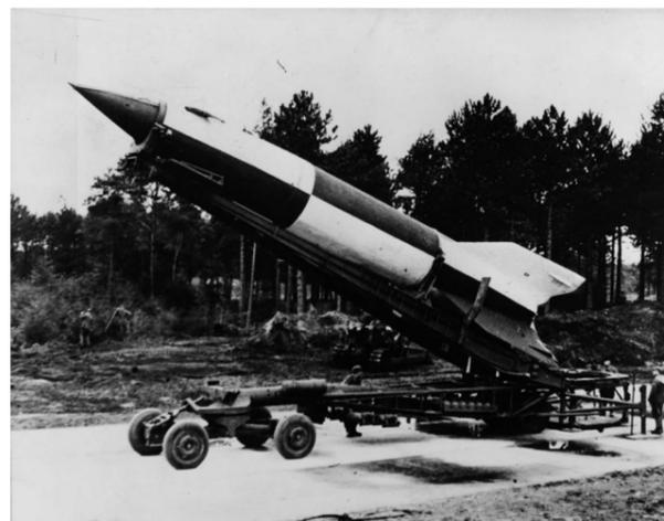
A V-2 rocket being erected for firing from its trailer, the „Meillerwagen“, near Cuxhaven in Lower Saxony. 1945.. Credit: NASA
