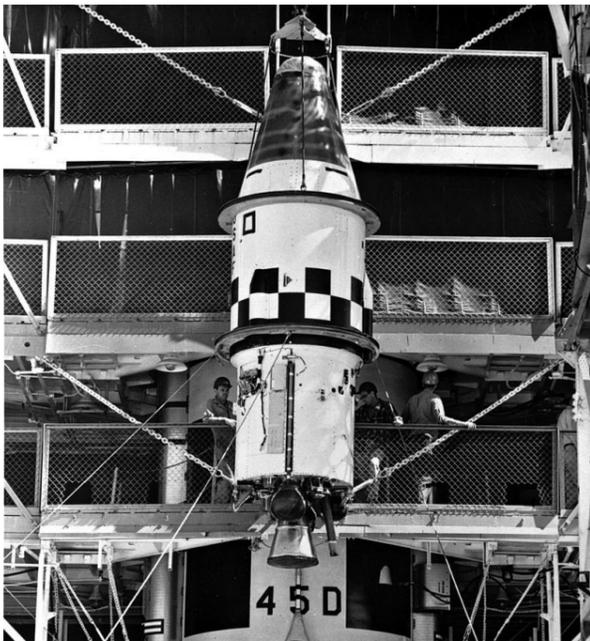
Agena A upper stage with Bell Model 8048 rocket positioned on top of an Atlas rocket at Cape Canaveral, ahead of the May 1960 launch of MIDAS-2
