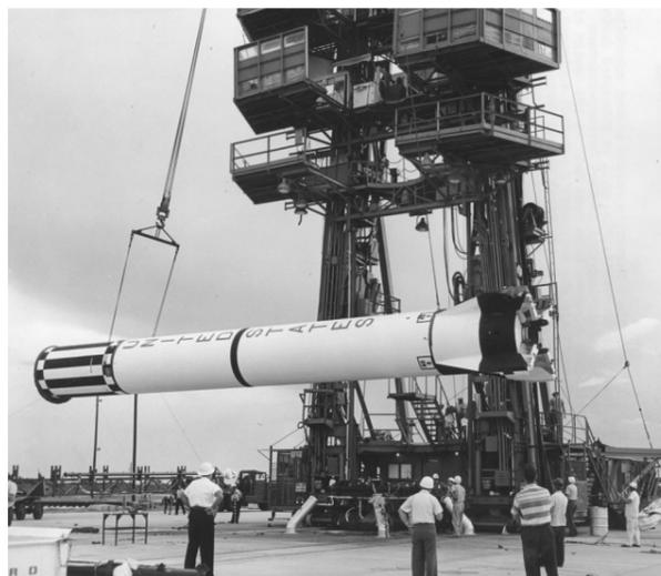
The Mercury-Redstone booster for flight Mercury-Redstone 4 (MR-4) is here being erected on the launch pad. Photo published on July 16, 1961, but probably taken much earlier, since the booster was normally erected weeks before the launch date.
